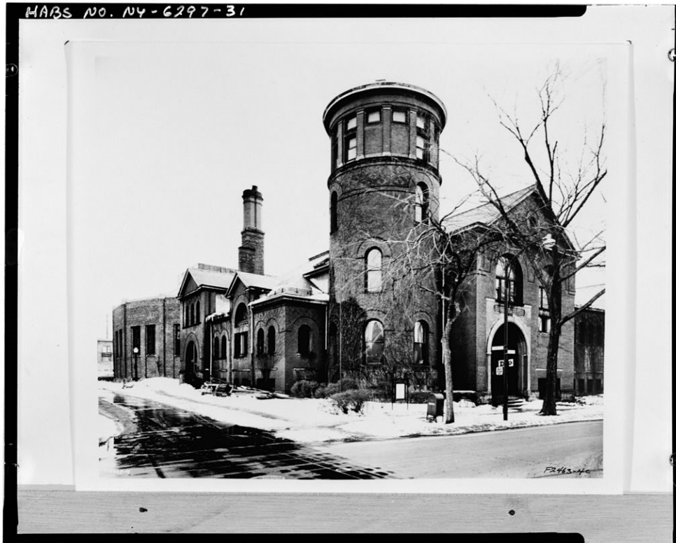
Figure 8: General view of building facing Southeast circa 1963.
