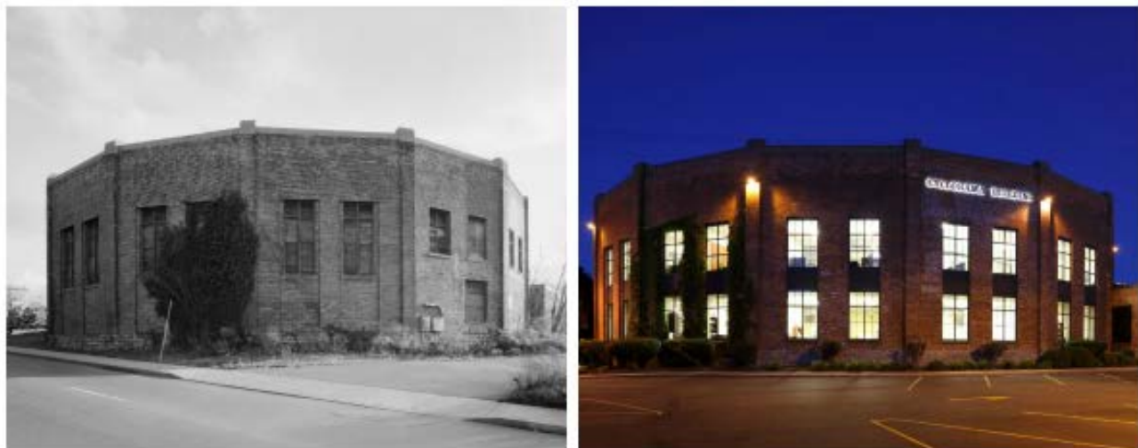
Figure 2: View of the Cyclorama building looking Southeast circa 1985, 2012.
